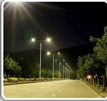
STREET LIGHTS & 24 HOURS ELECTRICITY
